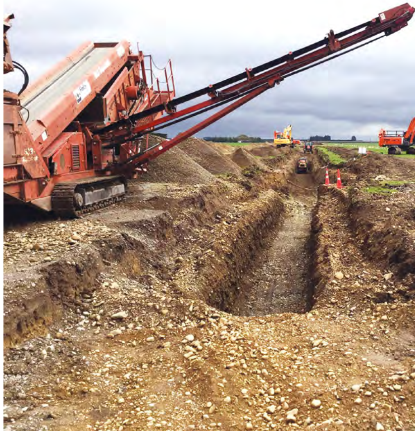
Ashburton-Lyndhurst Irrigation Scheme trench preparation for main pipe (1.28 m) installation
